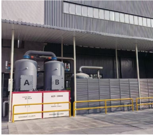
四川聯塑展開 PVC 主機抽濕羅茨真空泵組節能改造 Energy-Saving Upgrade of PVC Host Dehumidification Luoci Vacuum Pump System at Sichuan Lesso
